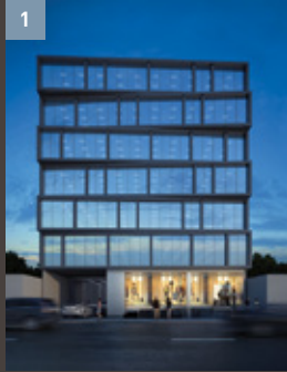
1 Of s Tower MIRAFLORES
